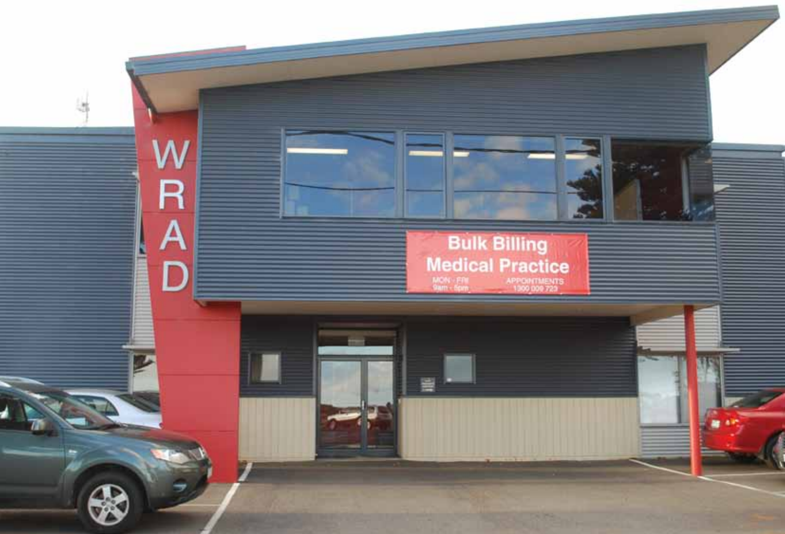
Pictured: The WRAD Building
